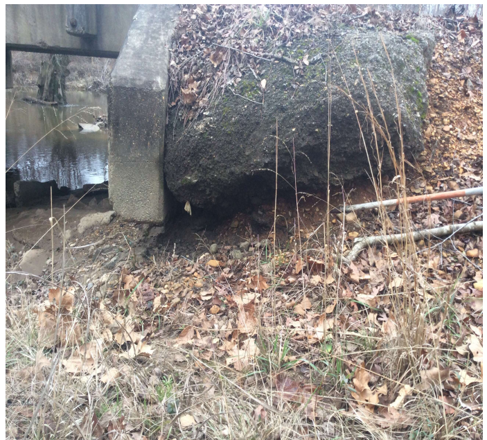
PHOTO 2 Description Abutment 1 left side scour under wing
