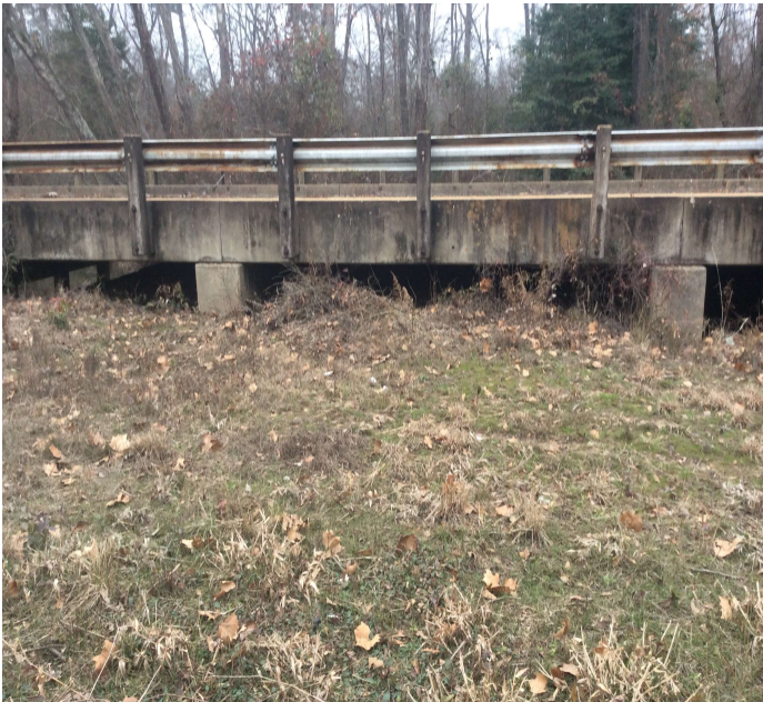
PHOTO 1 Description Spans 3,4 and 5 have severe degradation with 3 & 4 being the worst, thus this is causing the channel to scour abutment 1. There is little or no flow under spans 3 & 4.
