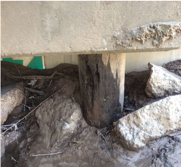
PHOTO 1 Description M0228 pile 1 bent 1 rotten with hole.
