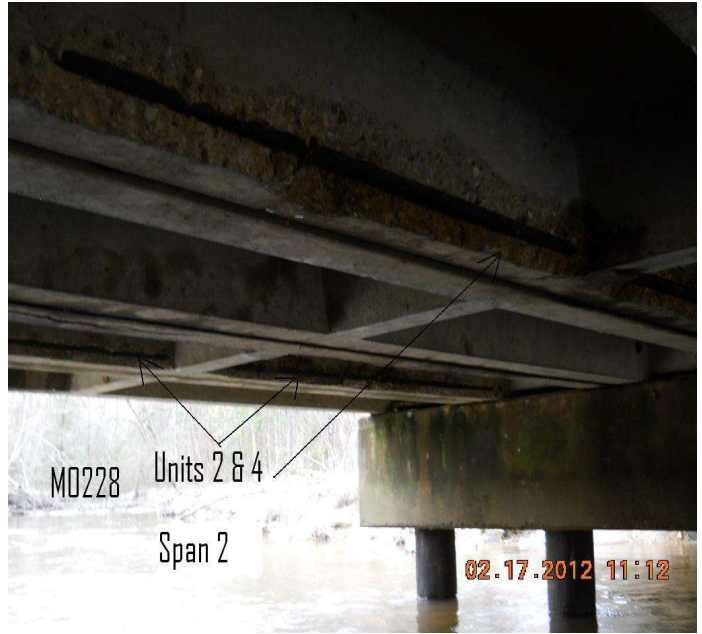
PHOTO 2 Description Span 2 PC units 2 & 4 have spalls with exposed steel.
