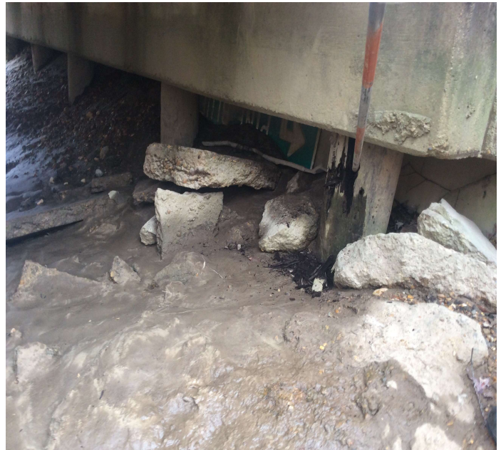
PHOTO 2 Description Pile 1 bent 1 rotten
