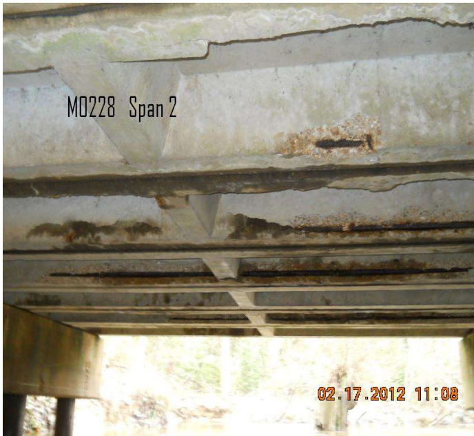
PHOTO 3 Description Span 2 PC units 2 - 5 with spalls and exposed steel.
