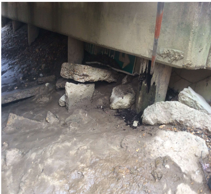
PHOTO 3 Description Abutment 1 scour back under the abutment.
